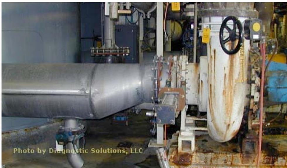
Figure 7.15 Pump suction with properly oriented eccentric reducer, well-developed suction flow profile
