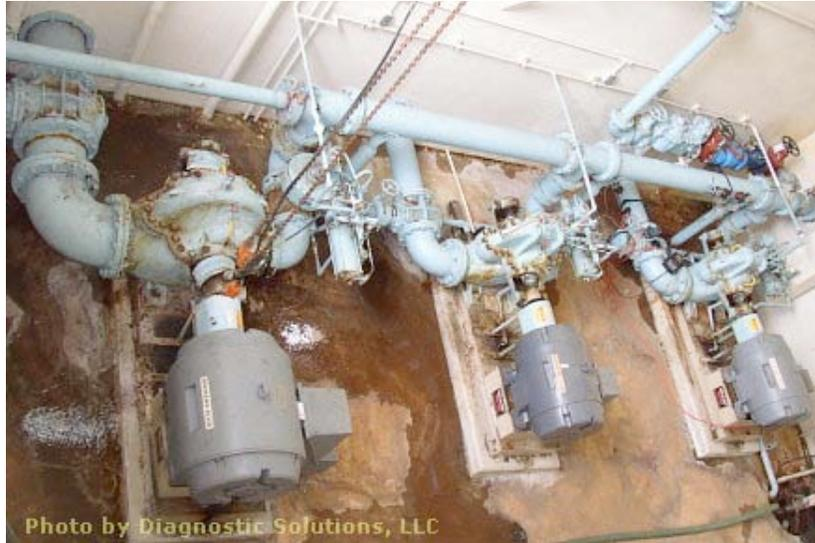
Figure 7.13 Pumping system layout with poor suction geometry (and little opportunity for improvement)
